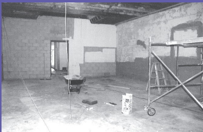
The back of the "new/future" Mobility Options enters the first phase of construction in late April.
